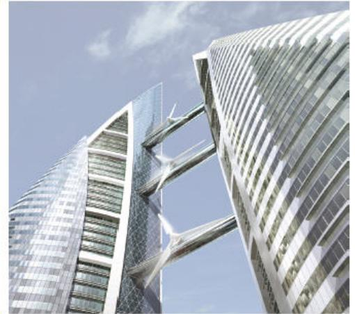
“The World’s first large-scale integration of wind turbines on a building.”
