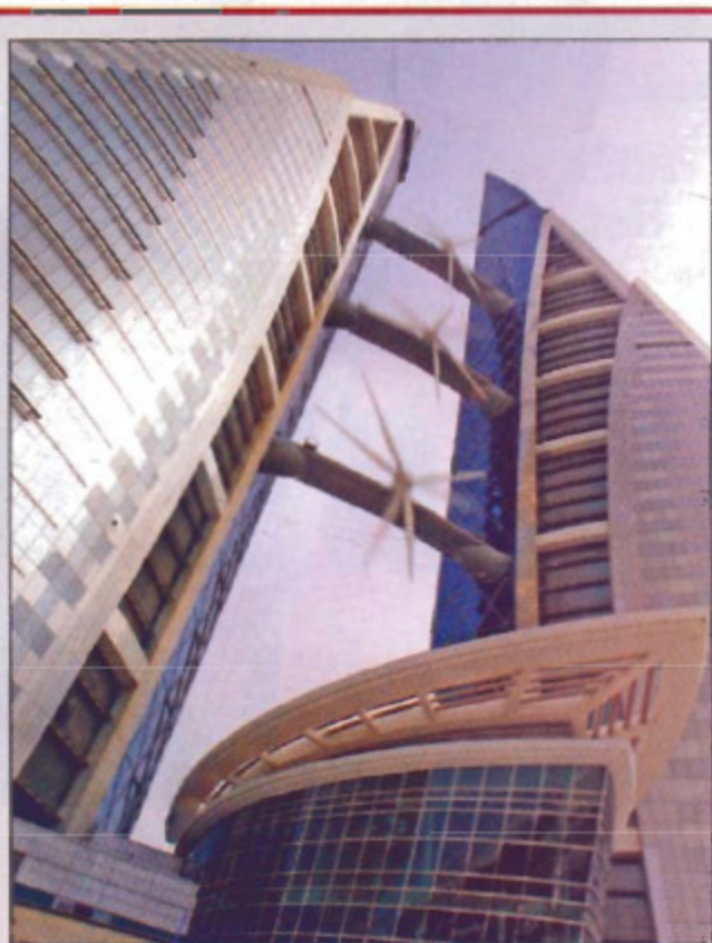
ANOTHER FIRST: The turbines in motion.
